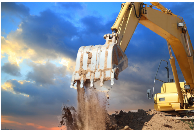
Figure 2. Key digital innovations are available for mines to keep workers safe and leverage increasing asset productivity.
