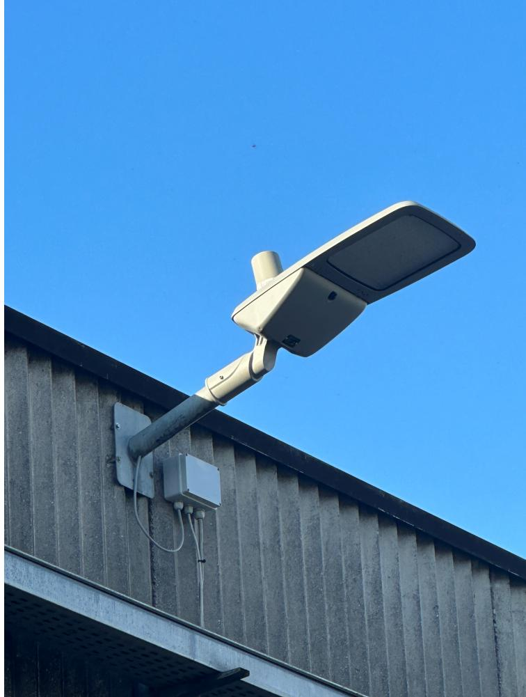
This is a lighting fixture with the sKy.Act LC mounted with Nema socket (the cylinder on top) to control the light. The box to the right contains the sGate and the Mesh node for connectivity. With this installation we can control the light scenarios and at the same time thanks to the sGate we participate into the infrastructure for the tracking.
