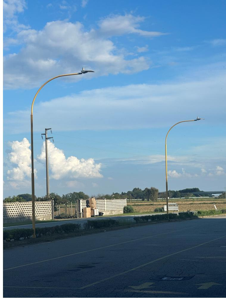
Lighting fixture with the sKy.Act LC mounted with Nema socket in the parking lot. Only Smart Lighting on this poles because in that area so far was not requested to have the tracking.
